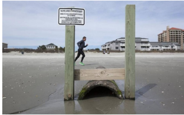
FIGURE 1.7: South Carolina stormdrain outfall and warning sign
