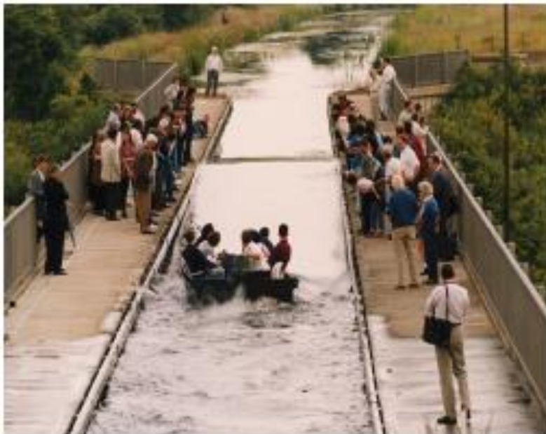
Figure1.2: Recreation of a solitary wave on the Scott Russell Aqueduct on the Union Canal. Photograph courtesy of Heriot-Watt University.
