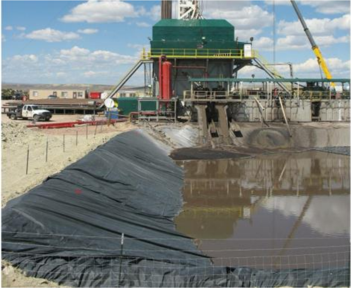
Figure 3.4: Reserve Pit Lined with Synthetic Liner (Ramirez, 2009).
